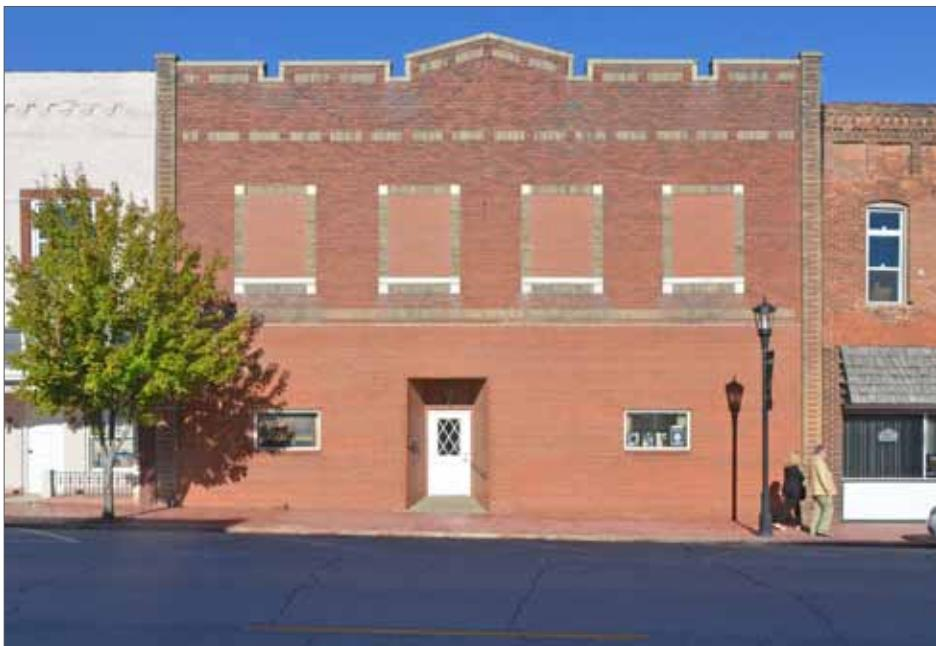
*Existing Conditions:* At some point in time, the storefront of this building was removed and/or bricked over. As a result, it offers no activity to the streetscape. Moreover, the door is of an incorrect style and the upper floor windows have been bricked in.
